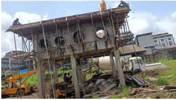
Photograph-20 Up-gradation works – DISTRIBUTION CHAMBER OF AERATION TANK
