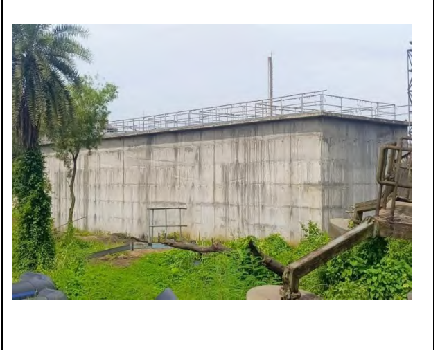
Photograph-18 Up-gradation Work- Anoxic Tank
