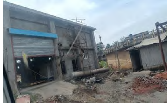
Photograph-21- Upgradation works – Blower House
